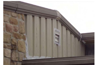
Sealant at Material Transitions
