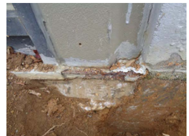
Metal Wall Panels at Grade
